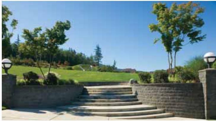
Maximum gravity wall height = 4 ft (1.2 m). Maximum reinforced wall height = 30 ft (9.1 m). Pisa2 units come in pairs and must be split on site. Please refer to the Pisa2 tech sheet for more detailed dimension information.
