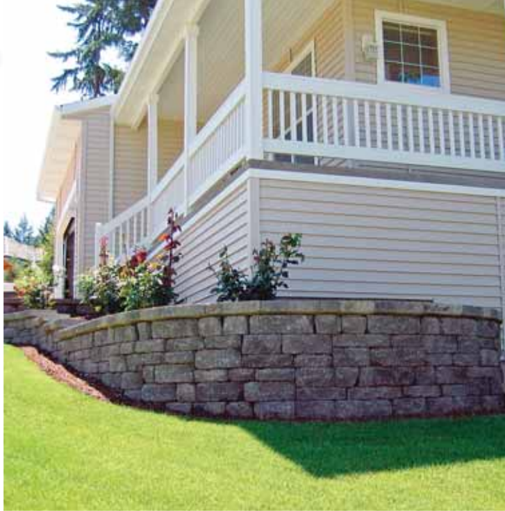
Maximum wall height = 21 in (0.53 m) for vertical walls, 42 in (1.06 m) for 8° battered walls. Please refer to the Celtik Wall tech sheet for more detailed dimension and design information.
