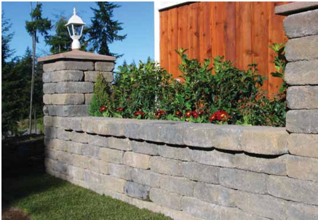
Maximum gravity wall height = 2 ft (0.61 m). Please refer to the TuscanStone tech sheet for more detailed dimension information.
